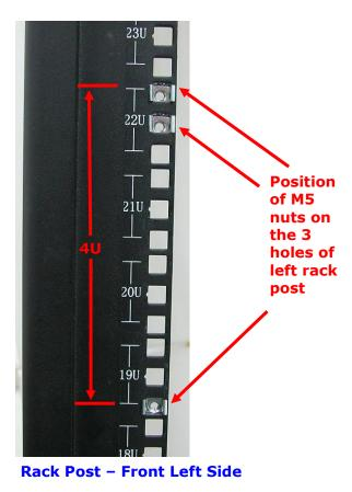
4. Insert three (3) M5 nuts on the 2 holes of the front right side of the rack post.
