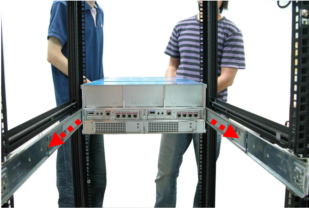
View from Rear Side
