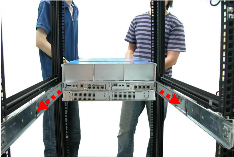
View from Rear Side
