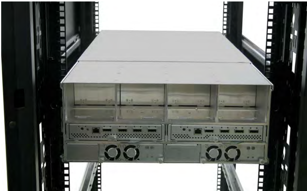
View from Rear Side of Rack Cabinet Enclosure is Pushed Inwards
