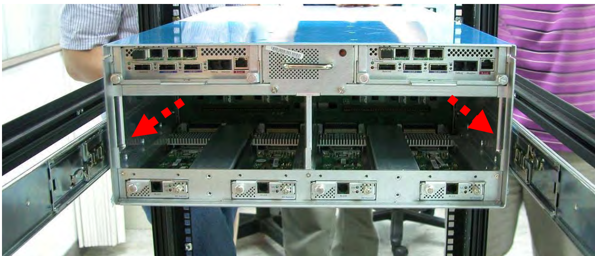
View from Rear Side of Rack Cabinet Enclosure is Pushed Inwards
